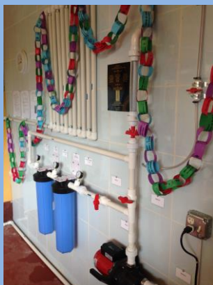
The completed clean water system
